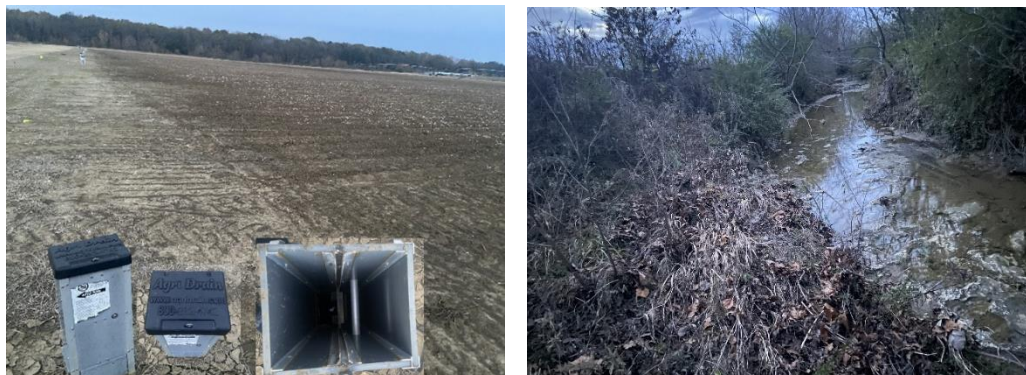
Fig. 8. Drainage system outlet at the edge of each of 16 plots and the outlet of the main pipes to the stream.
