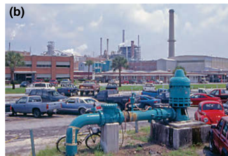
Large capacity well at a paper mill, St. Marys, Georgia. (Photo by Alan M. Cressler, USGS)
