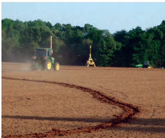
Photo 10-2. Surveying levees in a rice field.
